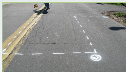
Typical survey paint markings
